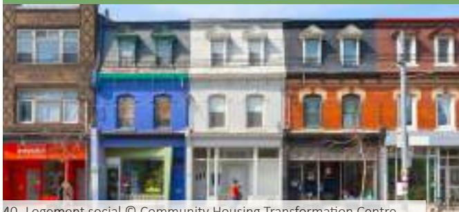
40- Logement social © Community Housing Transformation Centre
